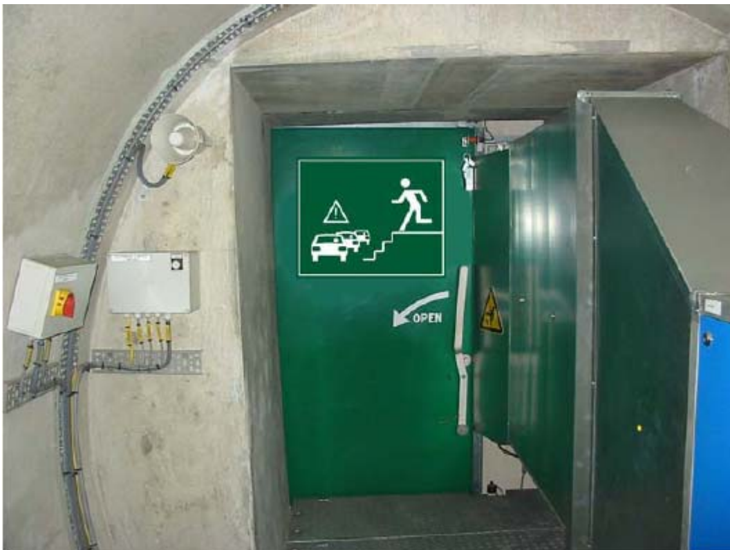
Figure 3: The TNO design to warn for traffic in the other tube.
